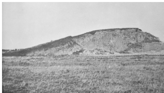
Fig. 11.: The damaged southern Török-halom kurgan in the 1970s (Dövényi et al. 1977, Fig. 7)
