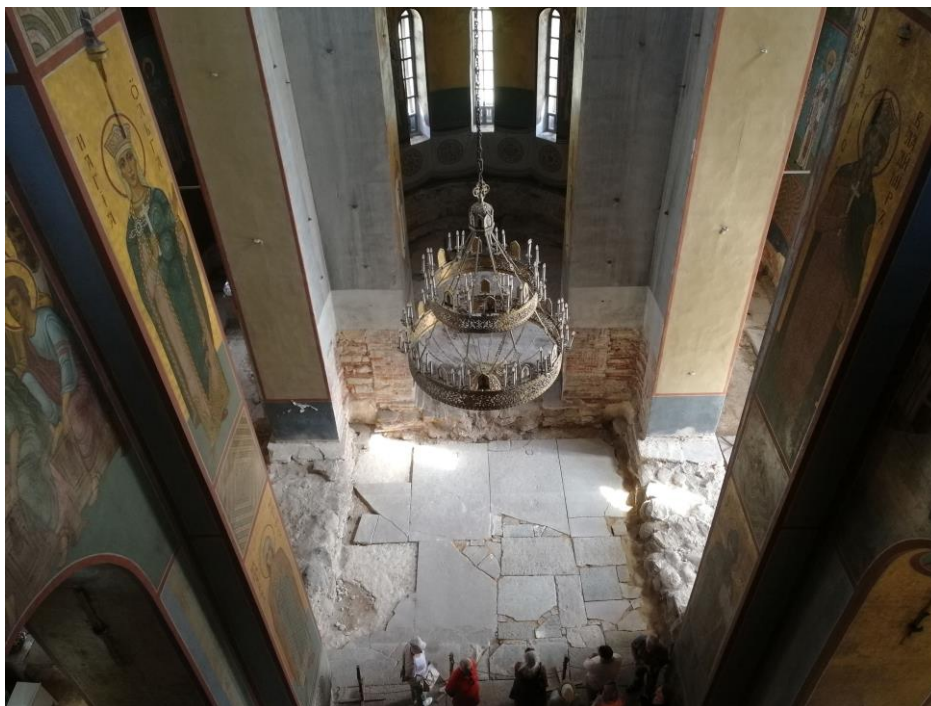
Fig. 2.: St. George Cathedral. Eastern part. Excavated constructions. View from Western gallery
